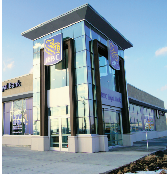
CORNICES & PORTAL ENTRY
